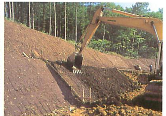
③ Restoration of topsoil 表土の張り付け
