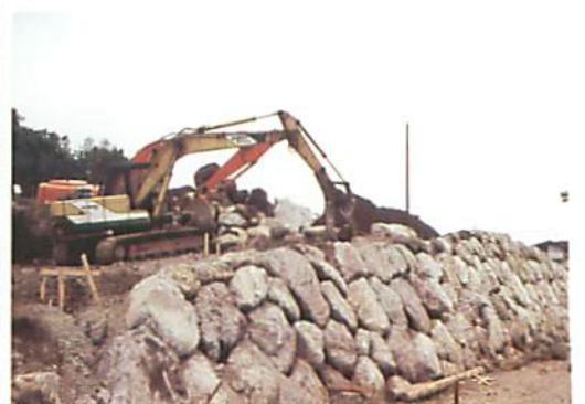
② Construction of retaining wall with stonework 巨石積みによる施工
