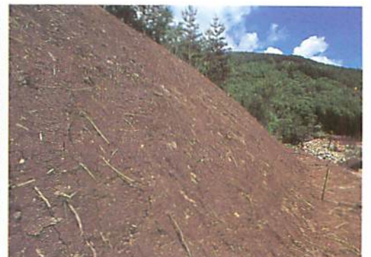
④ Topsoil restoration completed 表土復元の完了
