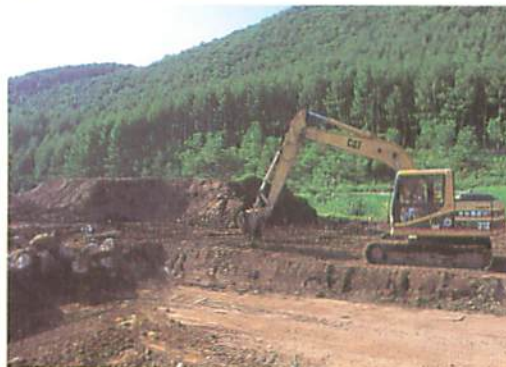
② Temporary settlement of topsoil 表土の仮置き
