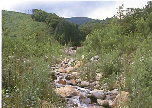
Channel modified for erosion control by ecological methods 自然環境に配慮された流路施工(白馬村)
