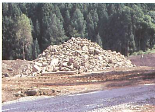
① Temporary settlement of stones 巨石の仮置き
