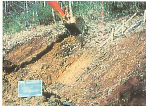
① Collection of topsoil 表土の採取
