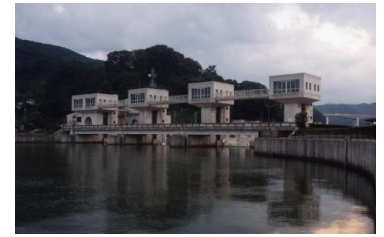
Current (2nd) "Kamaguchi Water Gate" Completed in 1988 (Maximum discharge 600m 3 /s)
